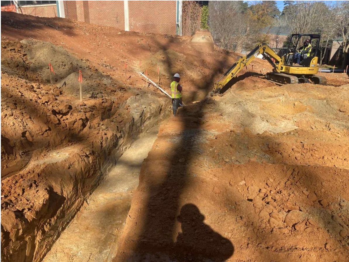
Cafeteria retaining wall footing install
