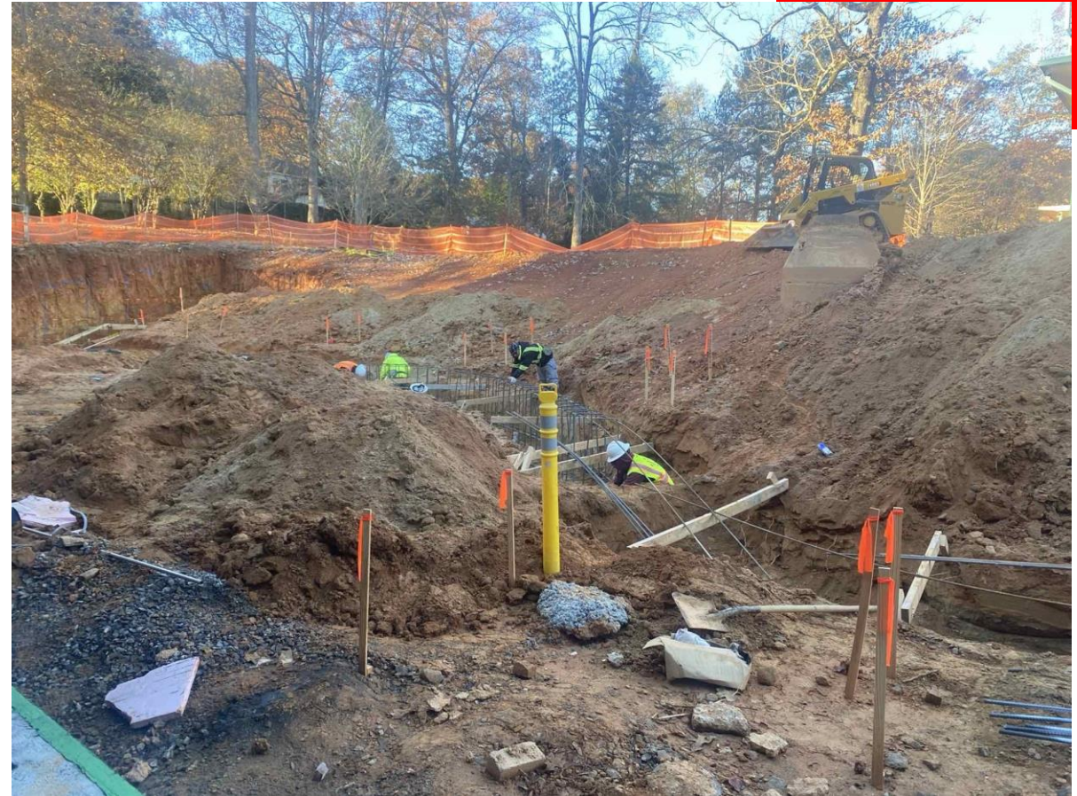
Cafeteria retaining wall footing install
