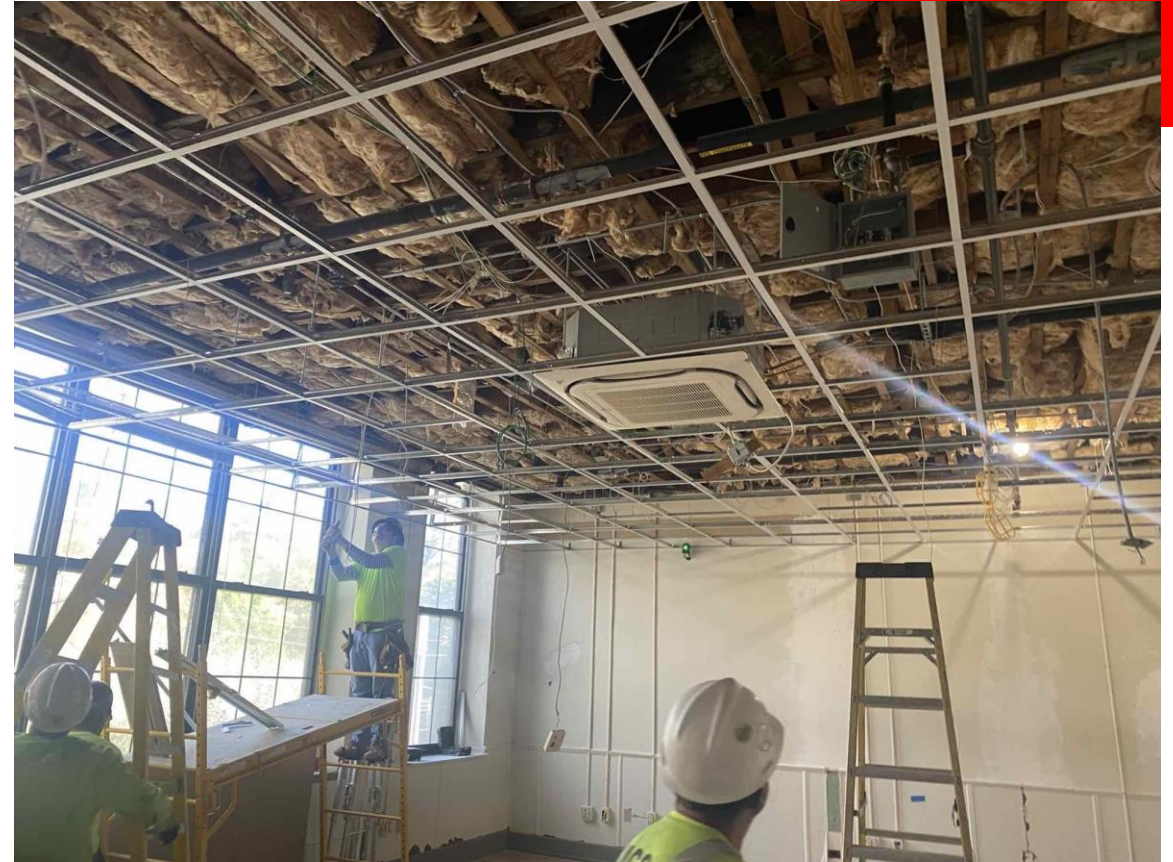
HVAC and ceiling grid install
